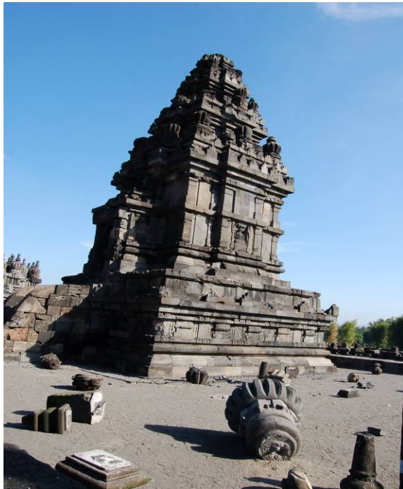
The Damage (Photo courtesy of BP3 DIY)
