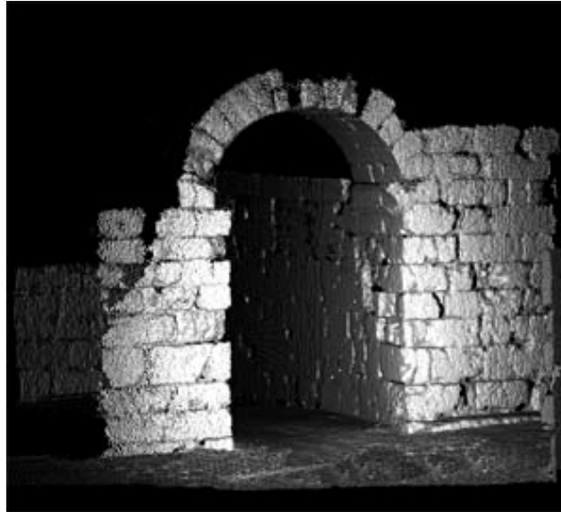
Cyrene, Theatre-Amphitheatre, the arch of access to the gallery north of the East Entrance: Texturing of the photographic image, carried out with 3D laser scanner, on a geometric model
