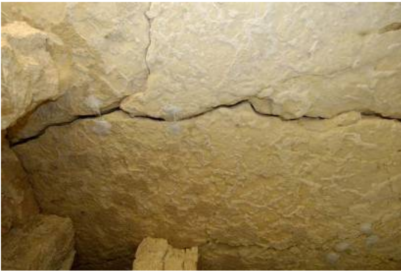
Cyrene, Theatre-Amphitheatre, hypogeum: view of the inner vault with the flaws and the glass “spies”
