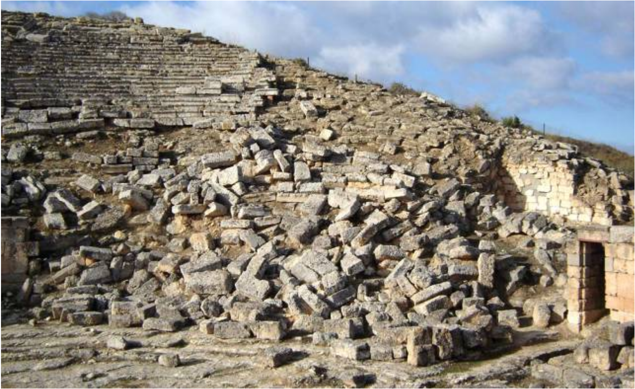
Cyrene, Theatre-Amphitheatre: the collapse of the west sector of the cavea
