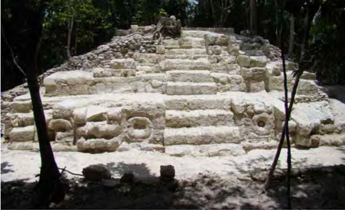
Above: Pava structure on first platform after stabilization and consolidation (Photo: R.D. Hansen).
