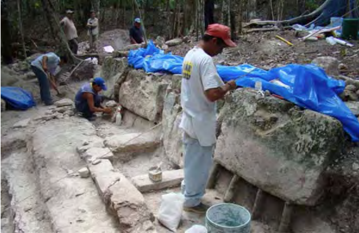
Above: Structure 304- Exposure and stabilization of massive monuments inset in the wall overlooking the great plaza to the north and located in the center line axis of the Central Acropolis. Additional data from excavations suggests that the platform was likely a royal throne (Photo: R.D. Hansen).
